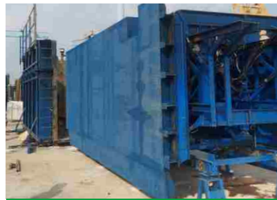
内模架 Internal formwork and framework
