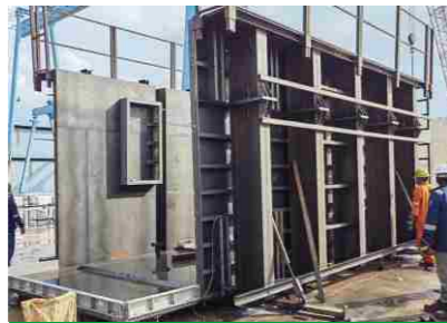
外模架 External formwork and framework
